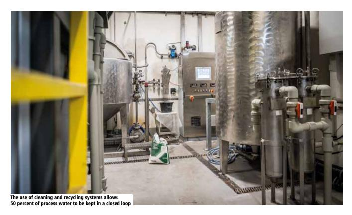
cleaning and recycling systems with a capacity of approx. 40 m<sup>3</sup>/h allows 50 percent of process water to be kept in a closed loop.
